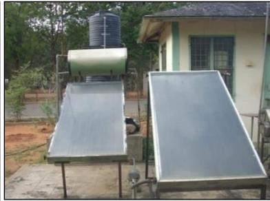
Solar Water Heater-Flat Plate Collector
